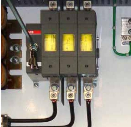
The Auto Deck staging conveyor has its own disconnect switch, but the fuse protection is handled inside the saw's main electrical enclosure with the same fuses used by the saw (shown in Figure 2-86). The Auto Deck's main enclosure is shown in Figure 2-87.
