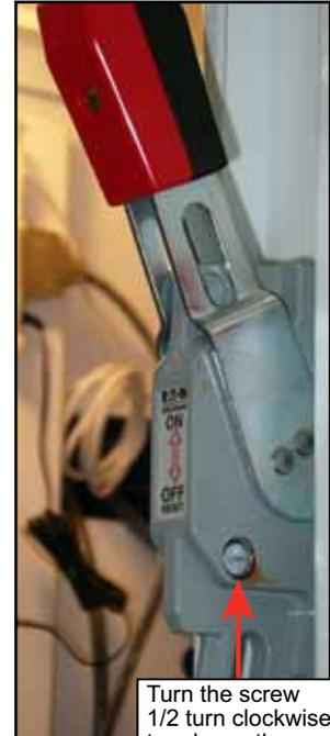
Turn the screw 1/2 turn clockwise to release the switch to open the door.
