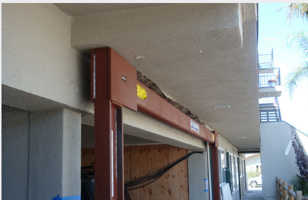
A Hardy Frame special moment frames was installed to protect this “soft story” garage opening. The special moment frame was painted to blend with the building.
