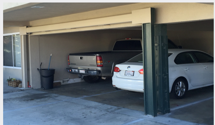
A Hardy Frame special moment frames was installed to protect this “soft story” garage opening. The special moment frame was painted to blend with the building.
