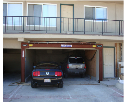
Hardy Frame special moment frames (SMFs) are designed to resist significant “inelastic deformation.” The SMF shown here can be specified in high Seismic Design Categories .
